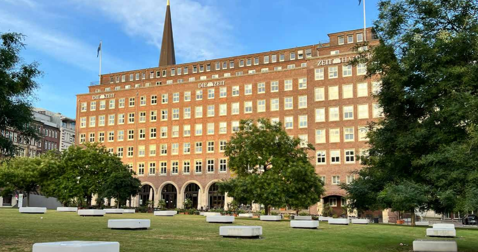
Headquarters in Hamburg, Germany
